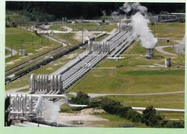
Geothermal power station, north of Lake Taupo, North Island. In this volcanic area, there is very hot water underground. When drilled, it gushes out as steam. This can be piped to a power station (above)
